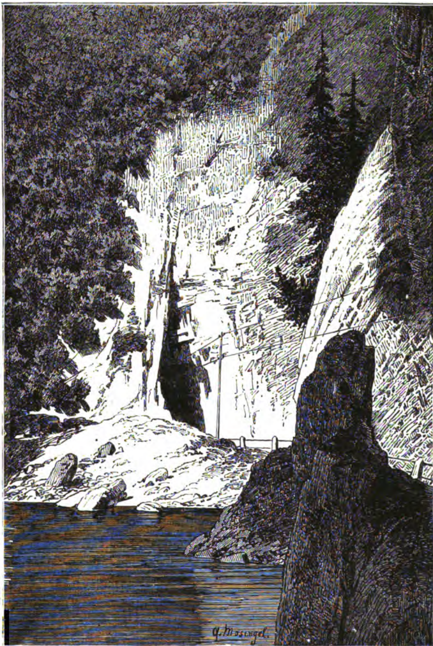
SOUTHERN ENTRANCE TO THE TUNNELS AND CUTS ON THE AXEN ROAD.
